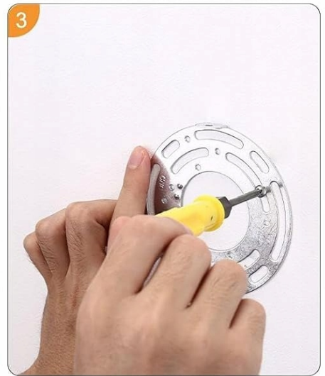
3 Use screws to fix the round stainless steel chassis to the wall
